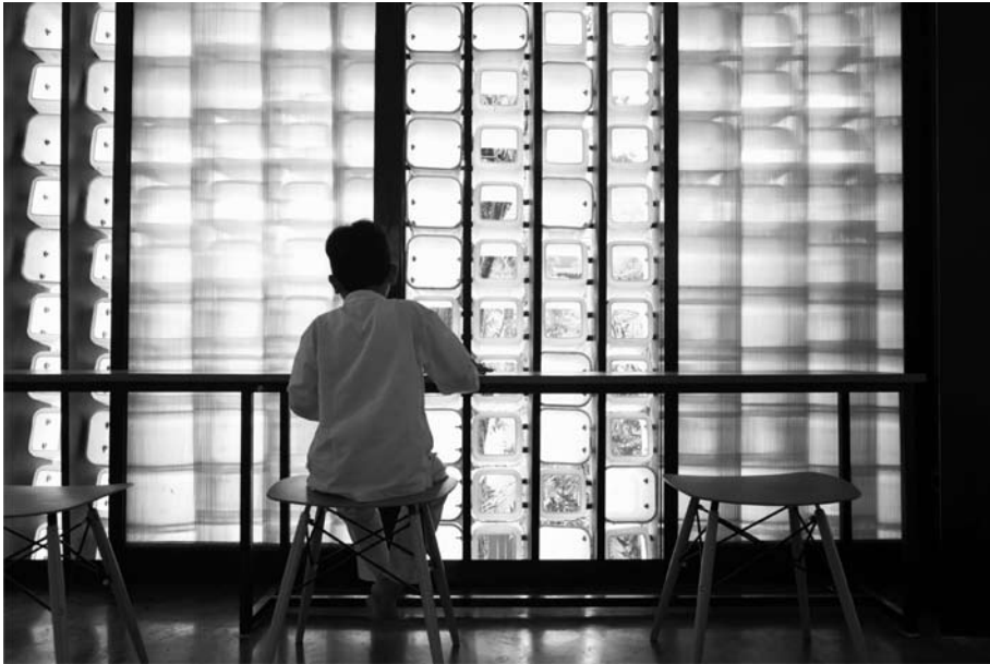
Fig. 2. Bucket façade seen from inside the Microlibrary, design by SHAU, photo by Sanrok Studio
