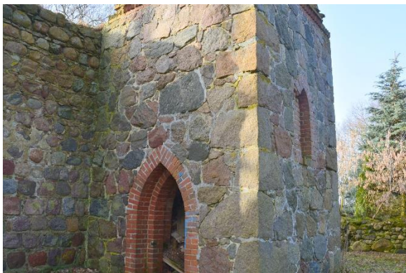
Fig. 8. Ruins of the church tower in Karwowo (photo by B. Cedro 2021)
